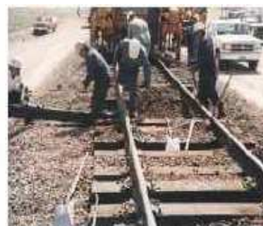
Recycled-plastic ties into test track
